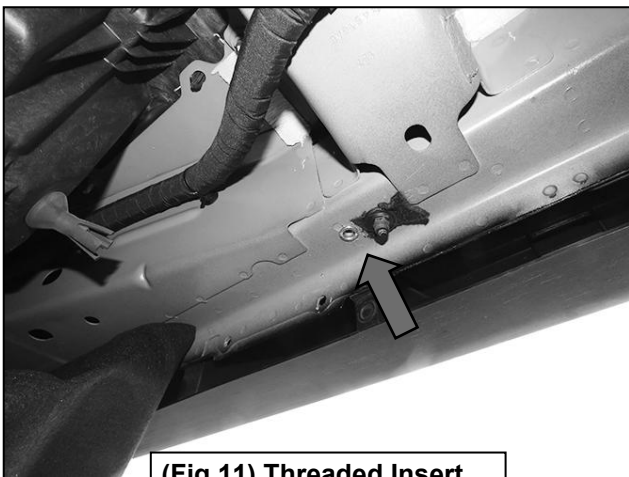
(Fig 11) Threaded Insert installed in the floor panel
