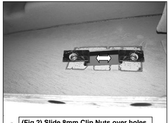
**(Fig 2)** Slide 8mm Clip Nuts over holes
