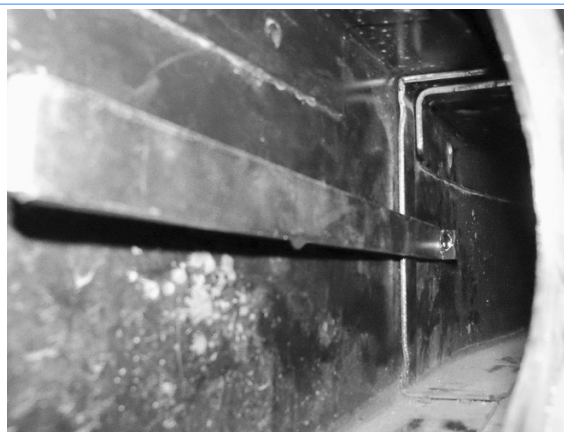
(Fig 3) M12 Long Bolt Plate Installed Inside View (In Frame Channel on Driver Side Front Mounting Location)
