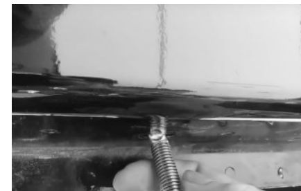
(Fig 3) M10 J-Bolt Installation (On Driver Side Mounting Location)
