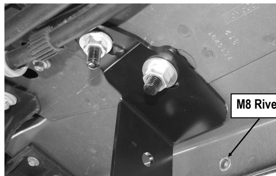
(Fig 17) M8 Rivet Nut Installed on Pinch Weld (Driver Rear Support Bracket Location)
