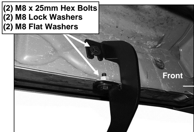
(Fig 6) Driver/left front bracket installed
