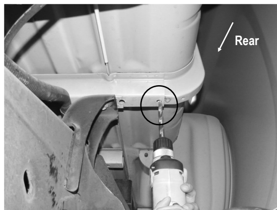
(Fig 15) Drill A 1/2" Hole Through The Channel
