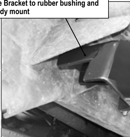
(Fig 3) Frame Bracket Installed
