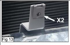
15. Take the two bottom extension brackets and install u-nuts onto the small ends aligning with the holes in the brackets (Fig 13) and oriented as shown.
