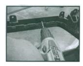
16. Drill a 3/16 inch holes for the mounting screws.
