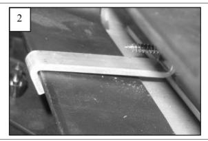
Center the grille in place. Wrap the hooks around plastic bars in the openings.
