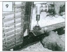
Install the side opening grille inserts. Install a screw from the front; secure a J hook and nut onto each screw. Center one of the inserts; Wrap the J hooks around the inner cross bar mesh. Tighten the hardware.
